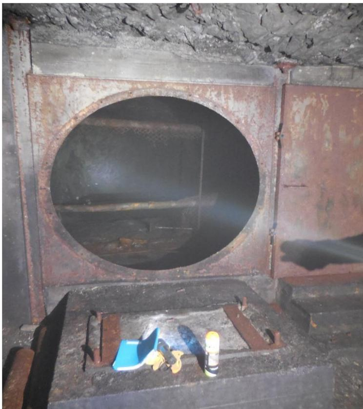
**Figure 3: Former location of a fan at the top of an air vent at level 1320**
