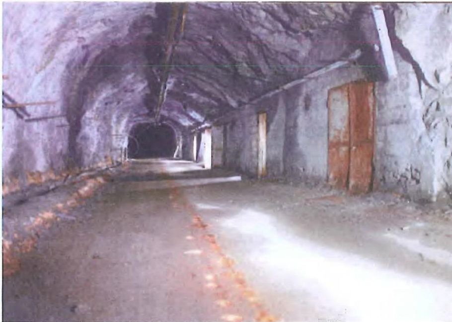
Figure 1: Mine access at level 1230 (Historical Photo)
