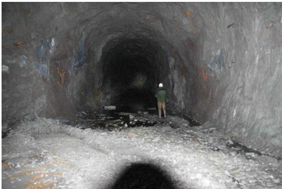
Figure 2: Mine development drive at level 1230 (Modern Photo)
